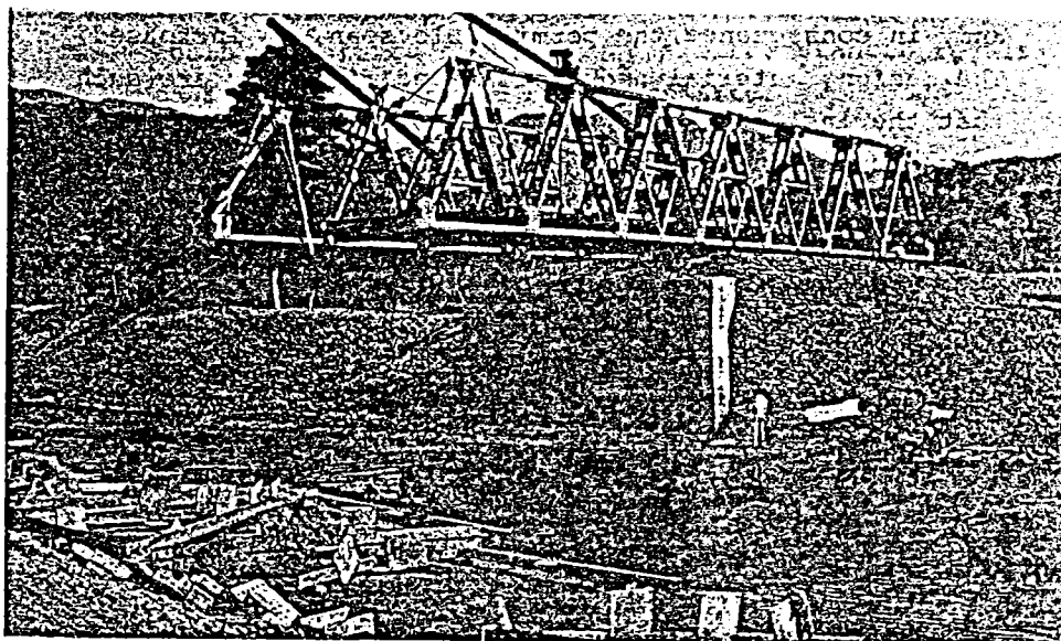
Photo 1 Cantilever erection of a Callender-Hamilton Type B15 Bridge in Nepal using basic erection equipment and local labour.
