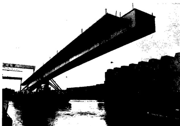
Fig. 8. Side span unit on barge ready to sail
