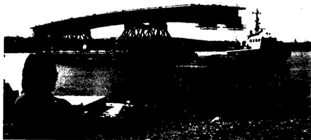
Fig. 20. Centre span units arriving at site for lifting
